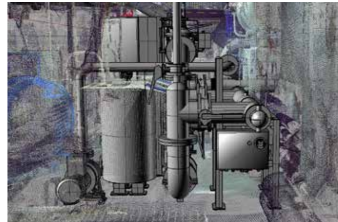
Ballast water treatment system modeled on 3D scan results.
