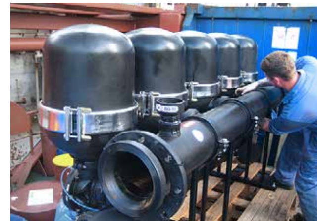
Goltens technician preparing a ballast water treatment system for installation.
