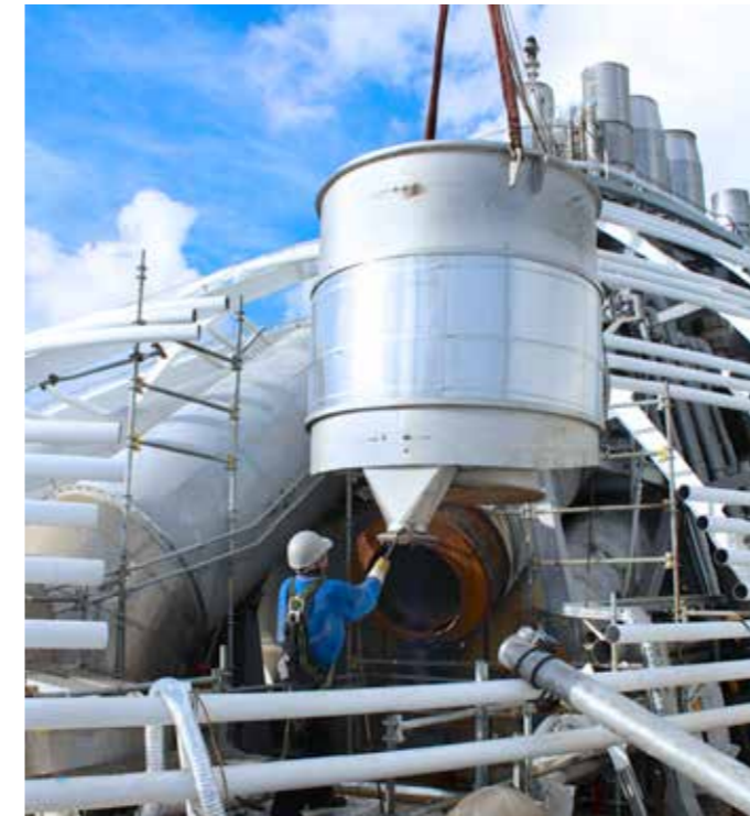
Rigging of new exhaust gas scrubber section aboard a cruise ship.
